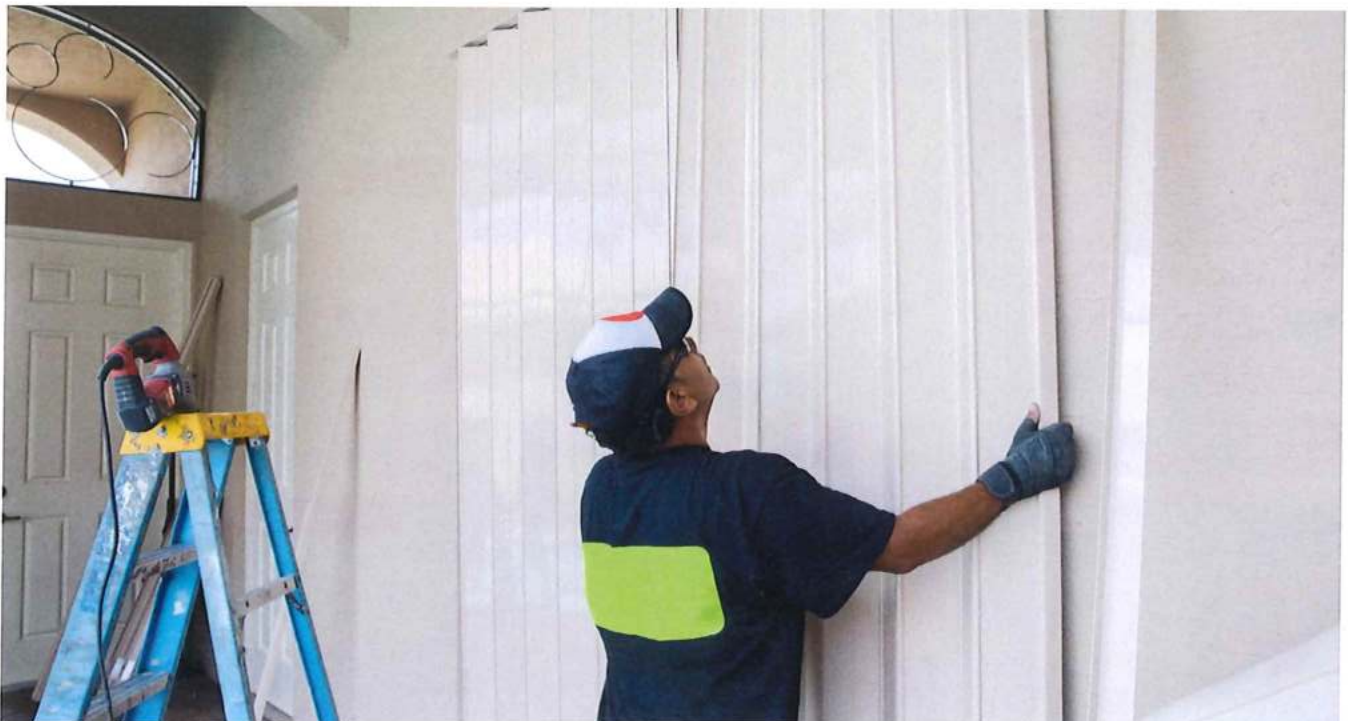
Photo description: Worker installing hurricane shutters inside a home.
